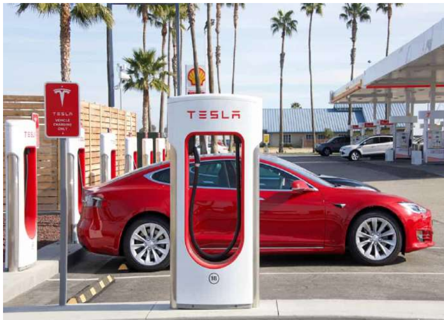
Figure 12: Tesla supercharger station
