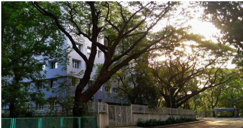
Fig 1.1 ESED Building, IIT Bombay
